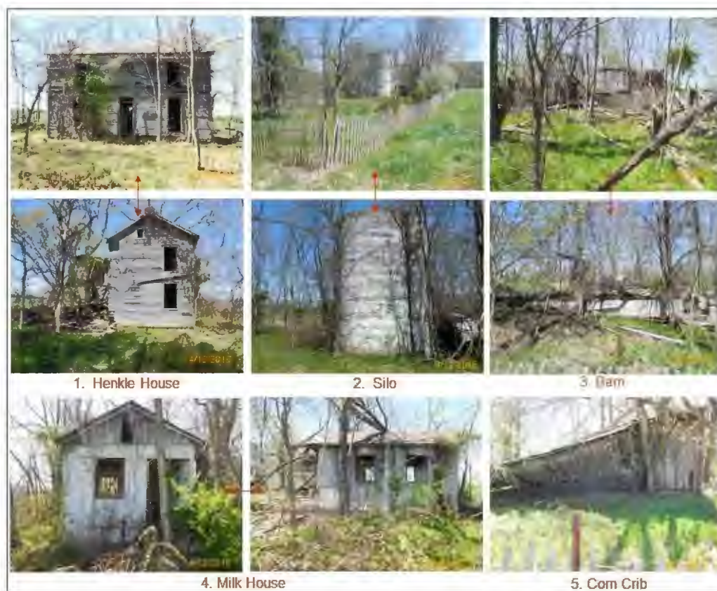
Figure 3: Photos of existing Henkle Farm House Structures
