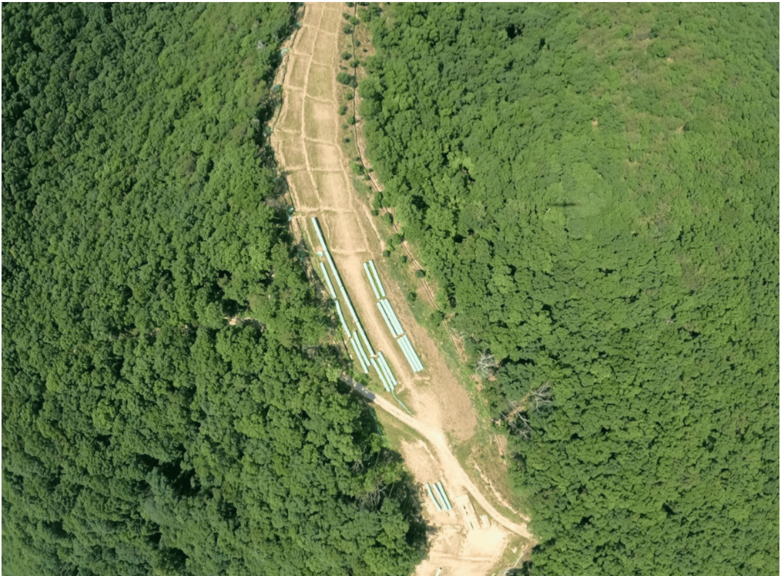
An aerial photo of the Mountain Valley Pipeline.
